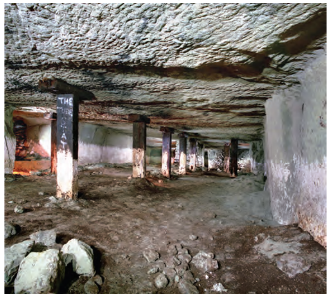
The remains of linear mushroom beds are seen here. The wooden props also date from this period. Photo Nick Catford
